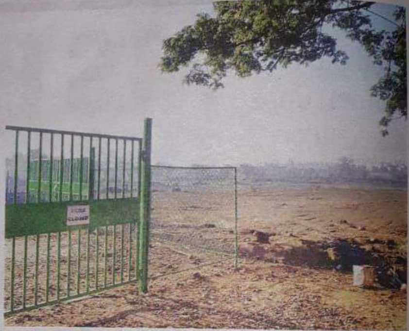
Though work on the Metro III project has been going on in full swing, the most debated proposal of removing 2,702 trees is on the cards now. REPRESENTATION PIC
